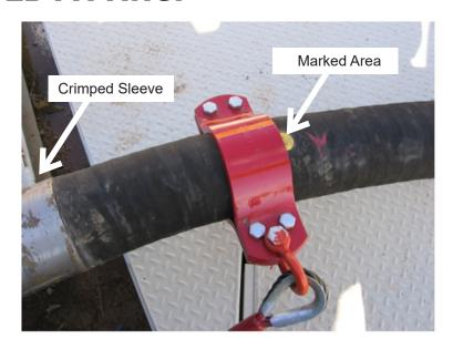
4 INSTALL HOBBLE CLAMP, TORQUE THE BOLTS TO APPROXIMATELY 60 FOOT POUNDS UNTIL CLAMP IS FIRMLY ATTACHED TO HOSE.
